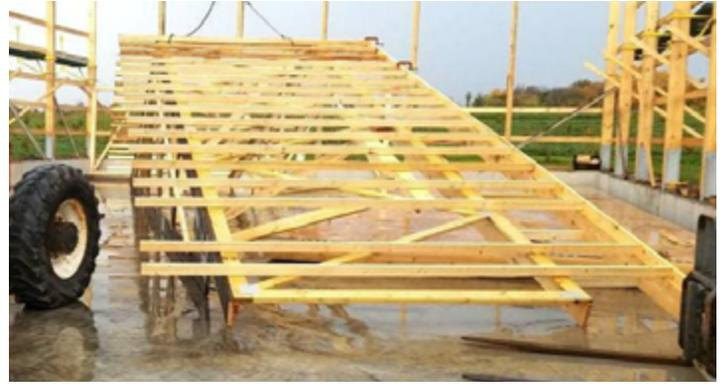
Figure 5. Ground assembly of a bay of roof framing that includes two diaphragm trusses (one on each side of the ridge).
