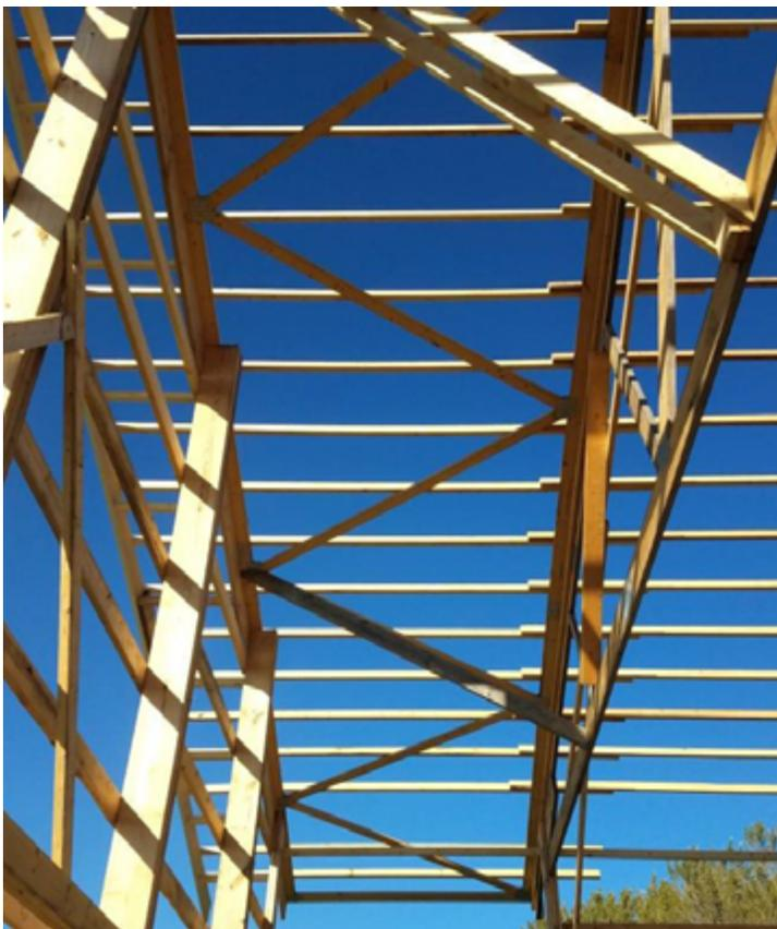
**Figure 2. Portion of a diaphragm truss in an end bay**
