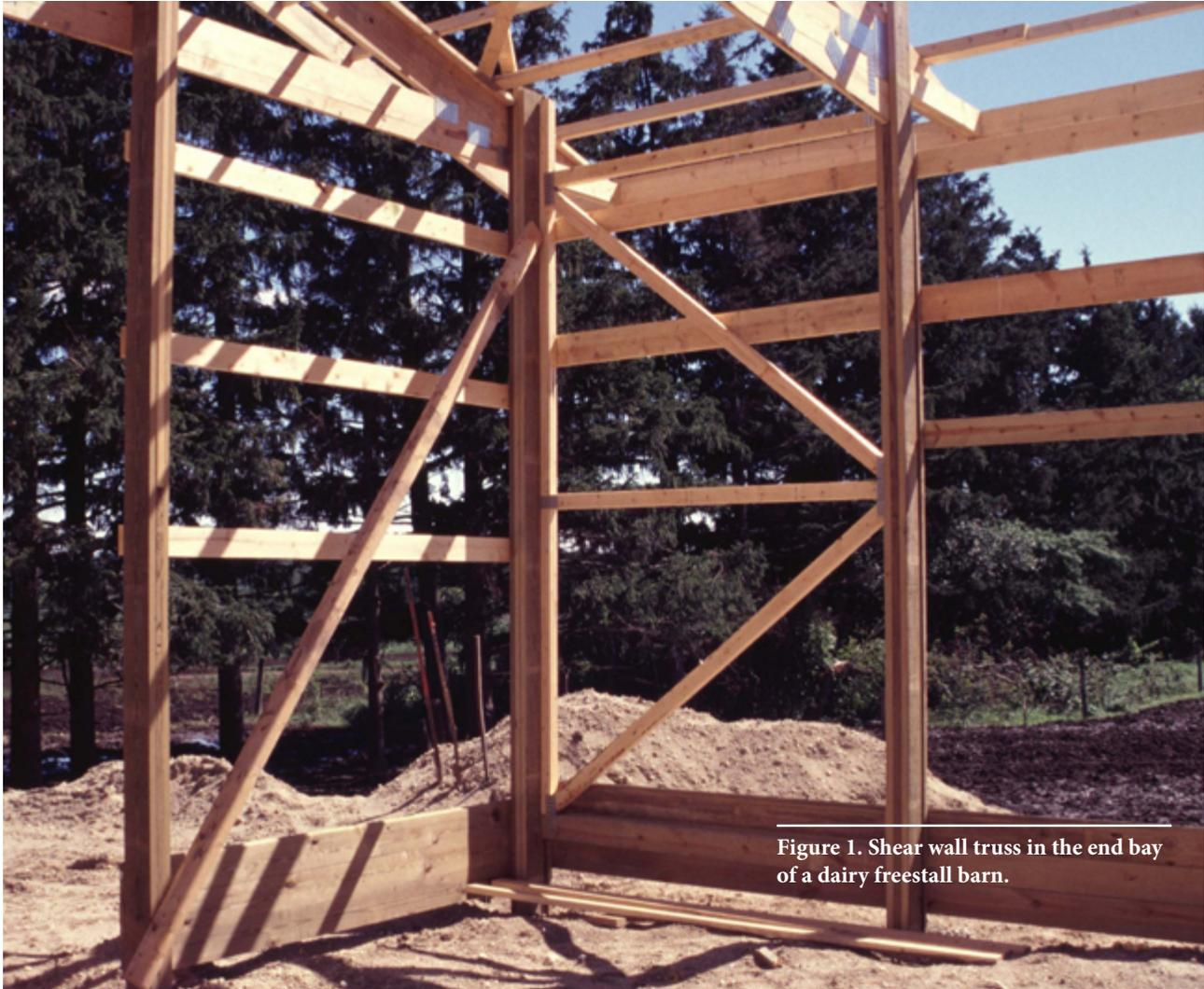
Figure 1. Shear wall truss in the end bay of a dairy freestall barn.
