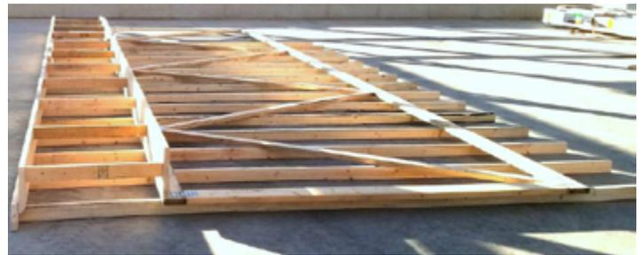
Figure 6. Diaphragm truss with attached purlins and rake overhang framing. Shown in an up-side-down position just prior placement.
