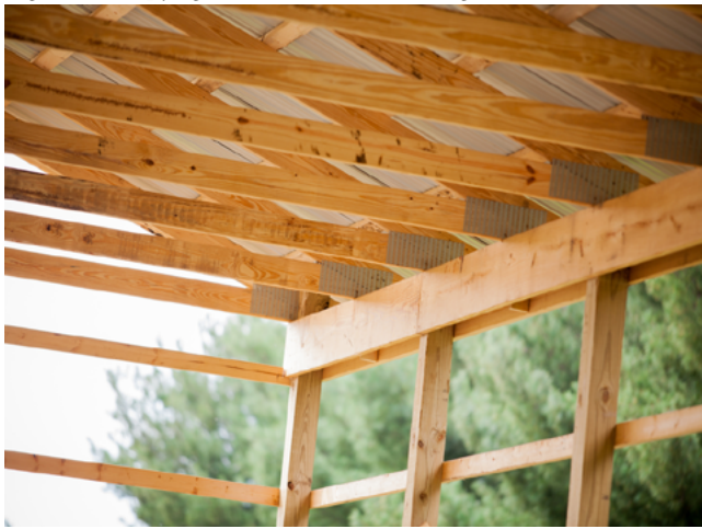
Figure 1. Copyright MilMar Pole Buildings
