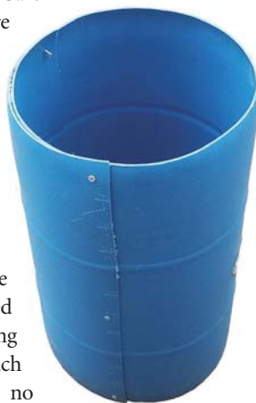
Figure 13. Pier form with 17.5-inch outside diameter (left) was fabricated from a used 55-gallon HDPE drum for insertion into a hole drilled with an 18-inch-diameter auger. Installed pier forms (center) were the sole vertical support for EFCO wall forms. Completed wall (right) features concrete-to-wood post brackets, exterior insulation, three runs of horizontal rebar and four vertical rebar that extend from the base of each pier to the above bracket. Concrete was simultaneously cast in pier and wall forms.
