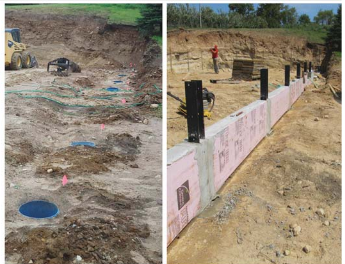
Figure 13. Pier form with 17.5-inch outside diameter (left) was fabricated from a used 55-gallon HDPE drum for insertion into a hole drilled with an 18-inch-diameter auger. Installed pier forms (center) were the sole vertical support for EFCO wall forms. Completed wall (right) features concrete-to-wood post brackets, exterior insulation, three runs of horizontal rebar and four vertical rebar that extend from the base of each pier to the above bracket. Concrete was simultaneously cast in pier and wall forms.
