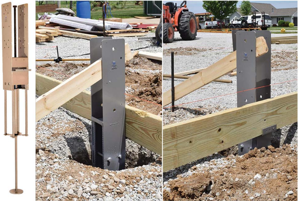
Figure 16. Strong Way Column features a vertically adjustable pier-to-post bracket (left) that vertically supports and is laterally supported by a splash plank during concrete placement.
