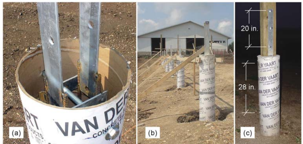
Figure 14. Post-to-concrete pier connection featuring straight side plates welded to steel reinforcing bars. Threaded rod with coupler nuts and bolts used to (a) fix bracket into place, (b) attach temporary wood braces to pier, and (c) provide anchoring points (at a 28-inch spacing) for steel partitions and gates.
