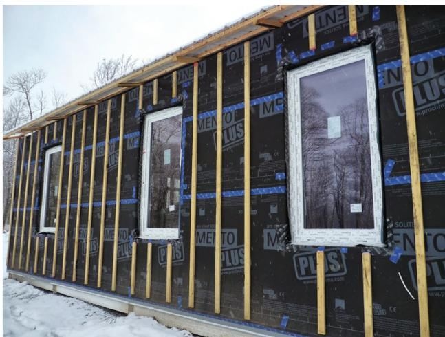
**Figure 16.** Project 3: Exterior view of wall framing and insulation system
