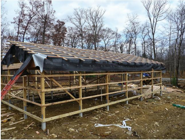
**Figure 14.** Project 3: Wall and roof framing during construction. Photos by Ben Freed.
