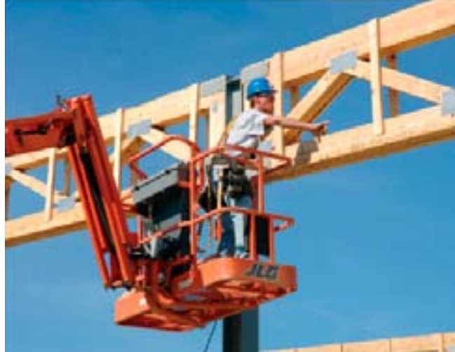
Figure 6. Worker using an aerial lift
