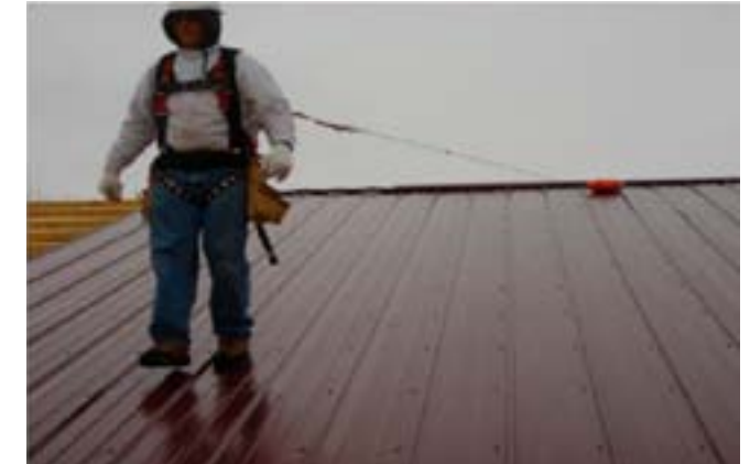
Figure 4. Worker using a single-point anchor
