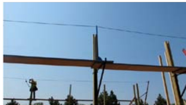
Figure 2. Horizontal lifeline used with a scaffolding system attached to posts
