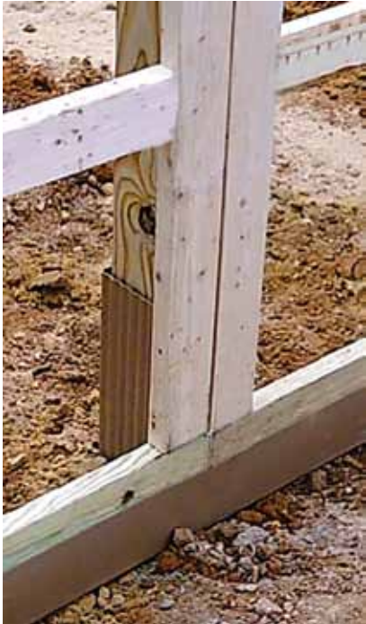
FIGURES 2a AND 2b. Plastic barrier system employing blow-molded HDPE 0.090-inch thick (Source: Ken McDonnell)
