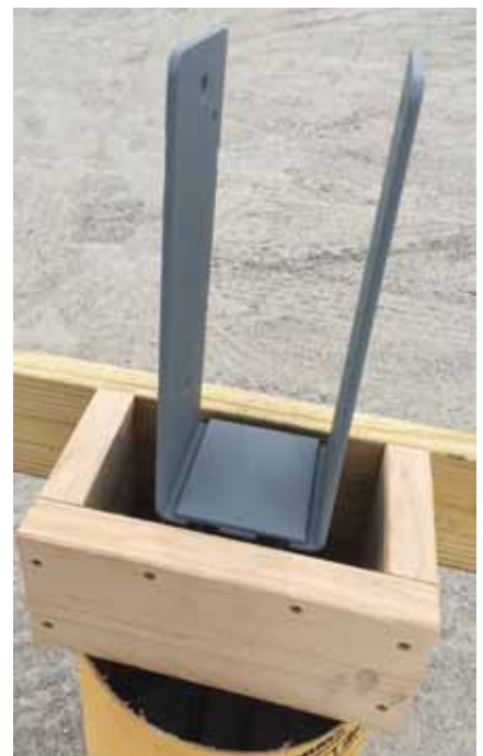
FIGURE 6. This cast-in-place pier uses a bracket that can either be wet-set into a form filled with fresh concrete or jugged in place for concrete to be poured underneath it. (Source: Brandon Meyer)
