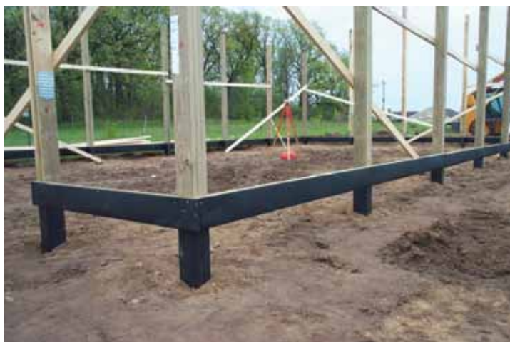
FIGURES 1a AND 1b. Plastic barrier system employing blow-molded high-density polyethylene 0.080-inch thick (Source: David Gruhlke)
