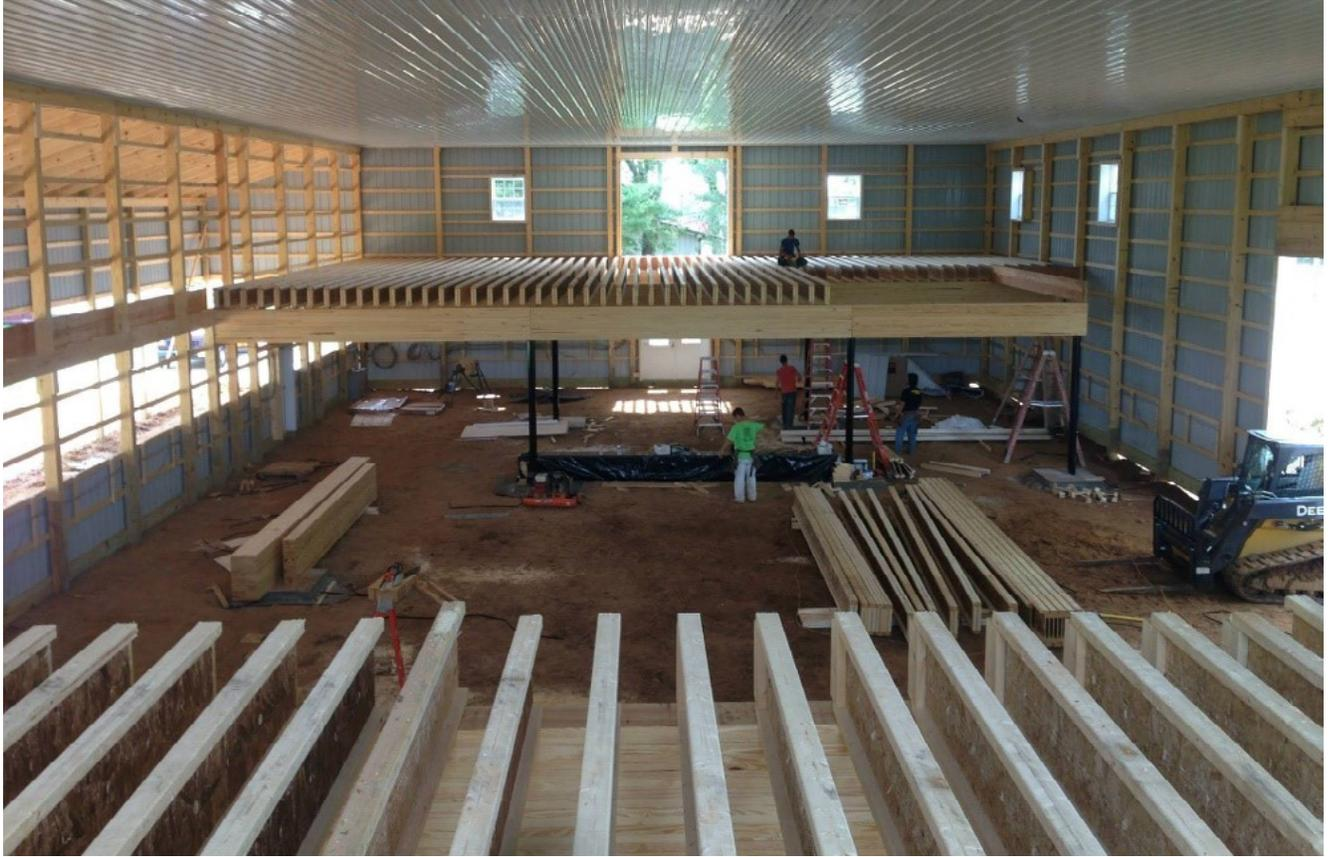
Example 1 Figure 2: View of glulam beams tied into building sidewall
