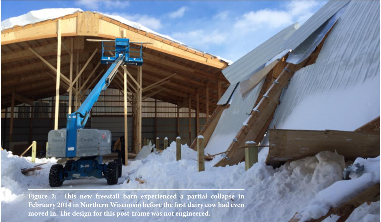
Figure 2: This new freestall barn experienced a partial collapse in February 2014 in Northern Wisconsin before the first dairy cow had even moved in. The design for this post-frame was not engineered.
