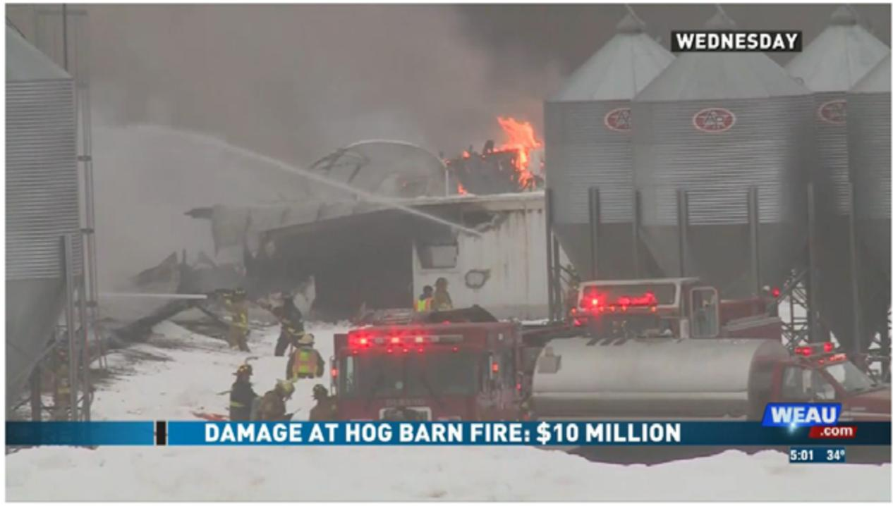
Figure 5: A post-frame hog barn collapsed in Wisconsin after a March 2019 snow event which then caught on fire from an electrical source. The building was engineered for a 30psf Roof Snow load, less than the ASCE 7 standard for the building's location.
