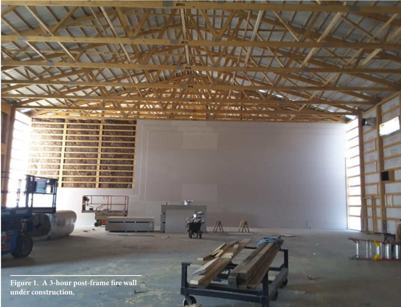
Figure 1. A 3-hour post-frame fire wall under construction.
