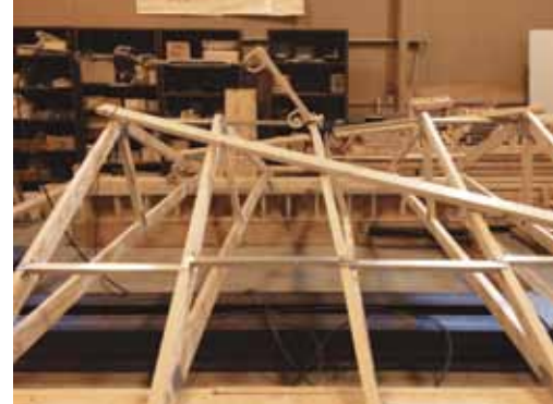
Figure 5. Loading of five-truss system with metal engineered bracing
