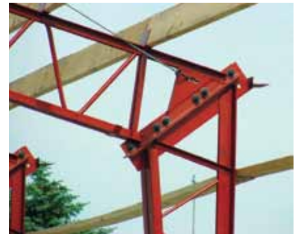
Figure 7. Rigid connection between steel trusses.
