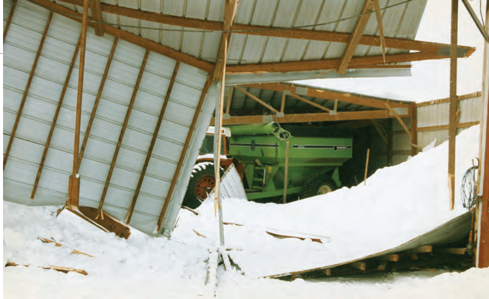
Top: The top of the end wall posts and gable were pulled into the building when the roof failed under the snow load. Middle: Roof failure caused the top of the wall posts to push out. Bottom: The knee braces slipped relative to post and truss chord, but did little damage to the wall as the roof failed under the snow load.
