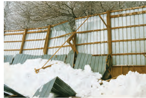
Top: The top of the end wall posts and gable were pulled into the building when the roof failed under the snow load. Middle: Roof failure caused the top of the wall posts to push out. Bottom: The knee braces slipped relative to post and truss chord, but did little damage to the wall as the roof failed under the snow load.
