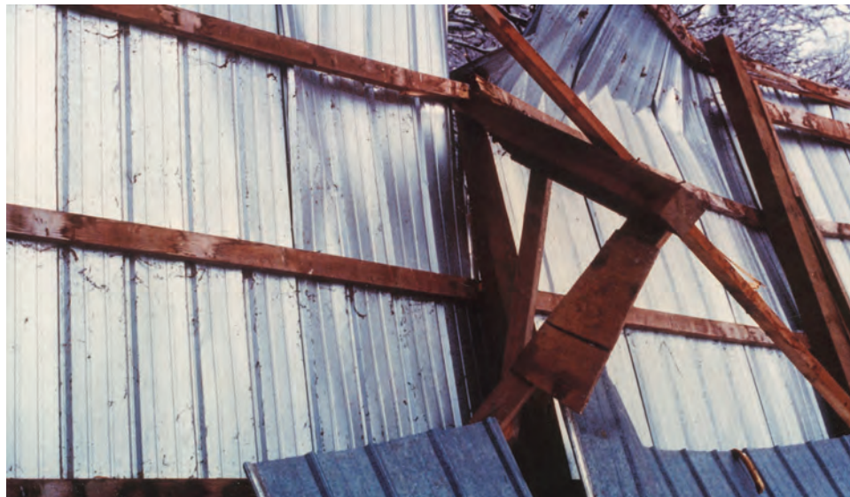
Top: The wall sheathing of this building was pushed out by knee braces due to snow load stress. Right: Roof failure under the snow load caused the wall posts to push out because the post-truss connection did not fail.
