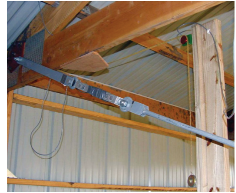
Figure 8. Eave displacement being measured with a washer-tensioned track attached to a rotary potentiometer, while force in a tie rod is measured with a specially constructed load cell.
