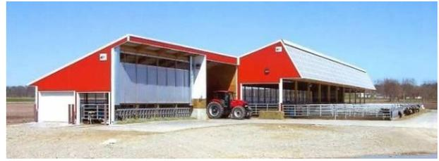
**Figure 1-47. Heifer growing facility with open sidewalls.**
