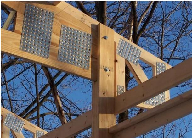
**Figure 1-55.** When truss is sandwiched between outer plies of a mechlam post, bolts are placed in double-shear for a very effective connection.
