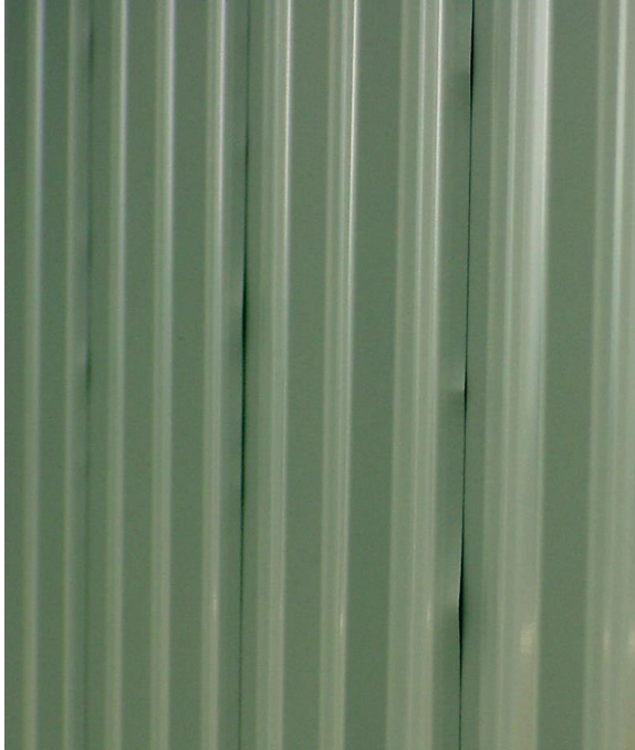
Figure 4 - Example of edge rippling. The middle wave in the right seam would be classified as an edge kink.
