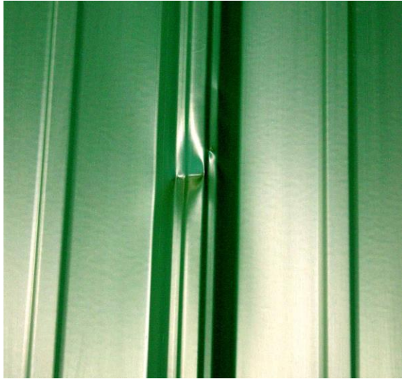
Figure 7 - Example of a rib kink.
