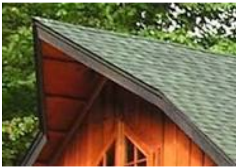
An extension of roof overhang extending at an angle to a peak beyond the normal overhang profile.
