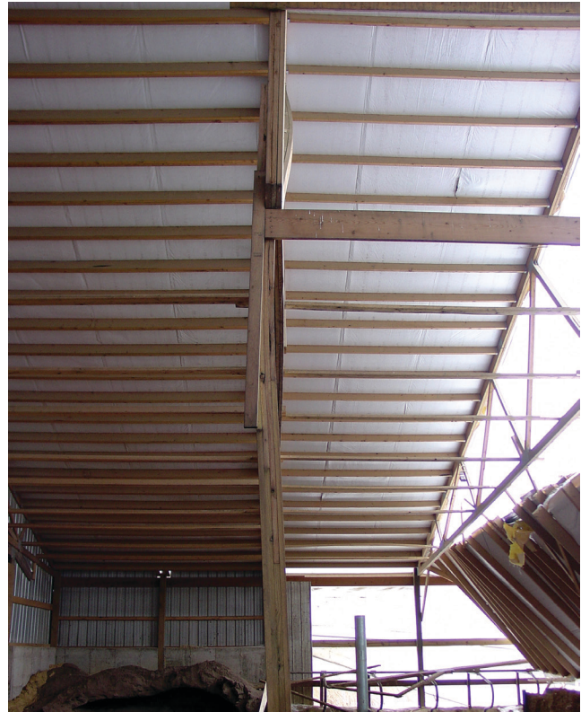
Figure 1: Buckling of a nail-laminated post due to improper design. Also visible is the buckling of the compression web chords due to improper bracing.
